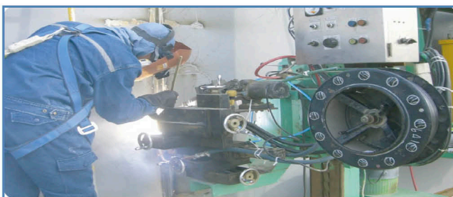
Vertical Automatic Welding
