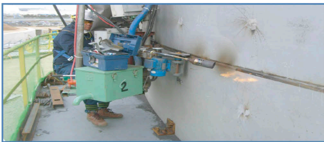
Horizontal Automatic Welding
