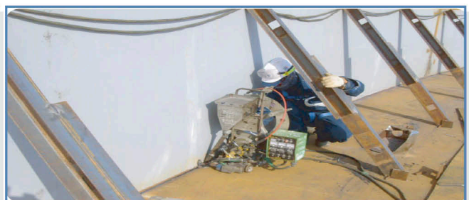
Corner Automatic Welding
